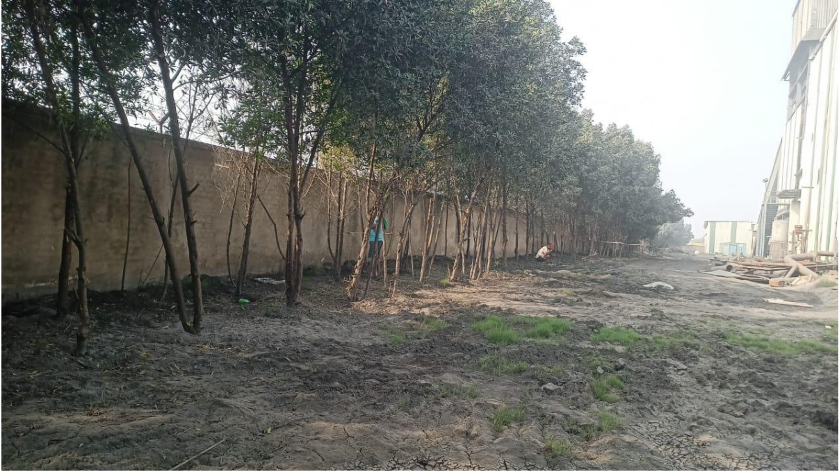
TURBINE AND BOILER AREA
